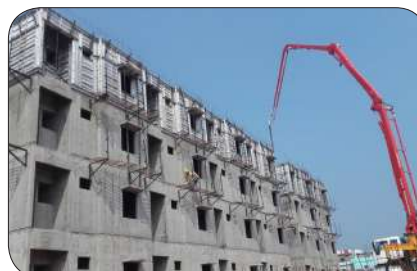
5. Monolithic Concrete Construction
